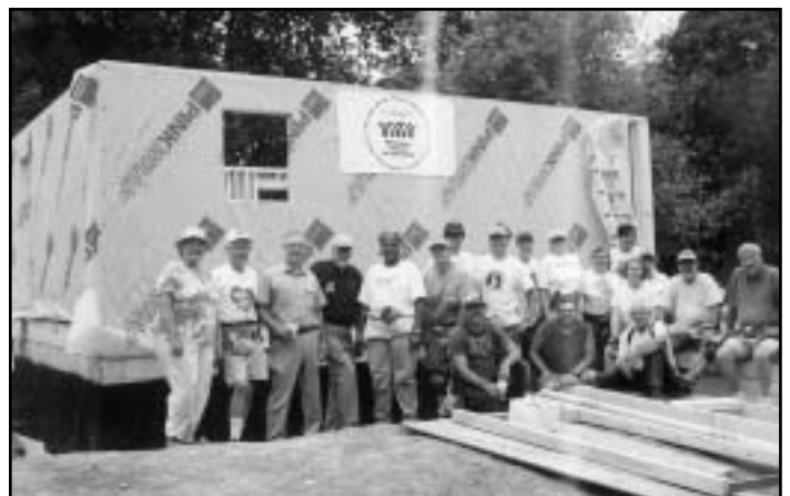
The Habitat for Humanity home being constructed by a team from SS. Peter and Paul and three other faith communities is getting close to completion now. The team gathered for a group picture when the walls were only partially built.
